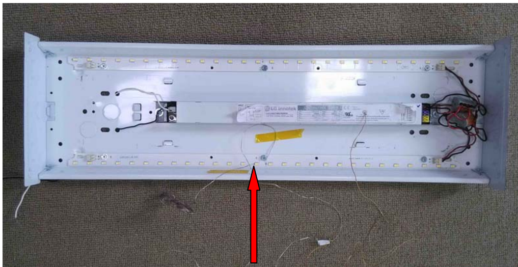
Location of In-Situ Point from overall view
