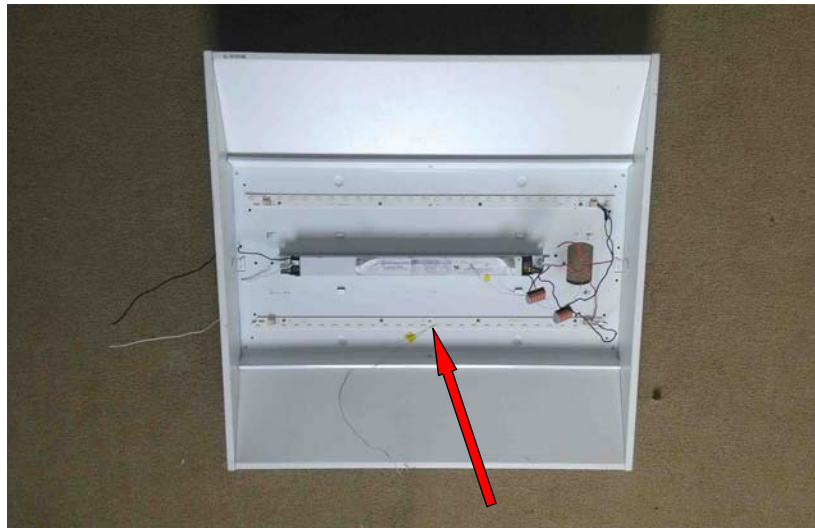
Location of In-Situ Point from overall view
